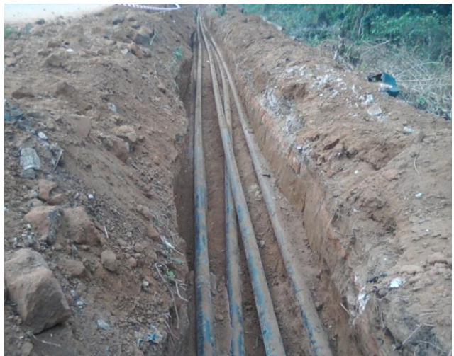
Repair / Sectional replacement of flowlines - SPDC
