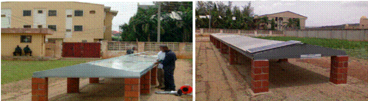
Installation of Tunnel Solar Dryer
