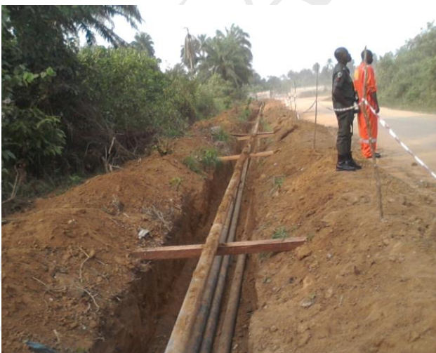
Repair / Sectional replacement of flowlines - SPDC
